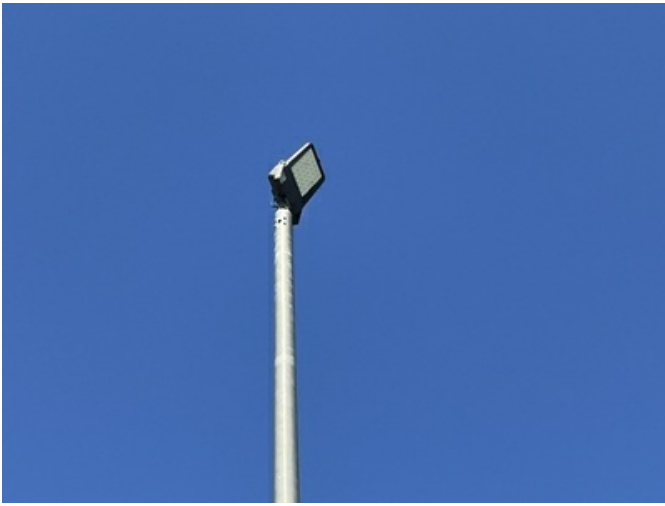
Light Pole in Required Area, Photo Taken by Joel Picou March 28, 2024
