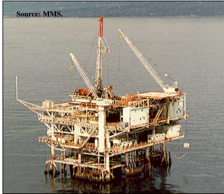
Figure E.3. Fixed Platform Structure.
