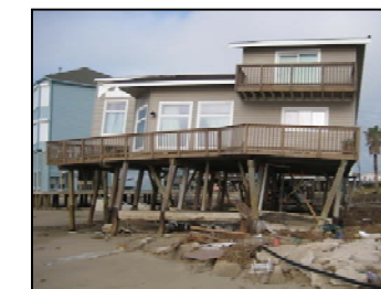
Fig. 2. Storm surge damaged to elevated houses on west end of Galveston Island during Hurricane Ike. Beachfront homes commonly experienced 1-3 feet of scour beneath the slab on grade. Left - Slab failure contributed to overall foundation failure of the structure. Right - although completely undermined - the slab remained intact, providing lateral bracing for the piles that saved the structure. Note the breakaway walls failed as they were designed to do.
