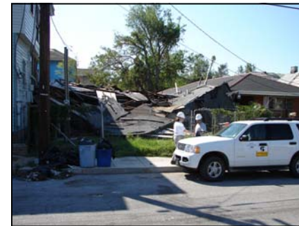
Carol Friedland investigating hurricane damage in New Orleans following Hurricane Katrina
