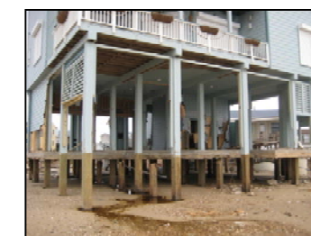
Fig. 2. Storm surge damaged to elevated houses on west end of Galveston Island during Hurricane Ike. Beachfront homes commonly experienced 1-3 feet of scour beneath the slab on grade. Left - Slab failure contributed to overall foundation failure of the structure. Right - although completely undermined - the slab remained intact, providing lateral bracing for the piles that saved the structure. Note the breakaway walls failed as they were designed to do.
