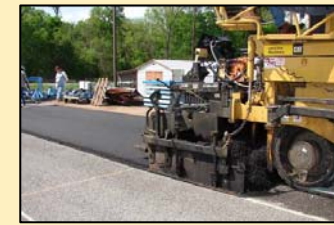
FIGURE 4 Spraying of Tack Coat and HMA Overlay Construction
