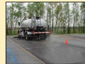
FIGURE 4 Spraying of Tack Coat and HMA Overlay Construction
