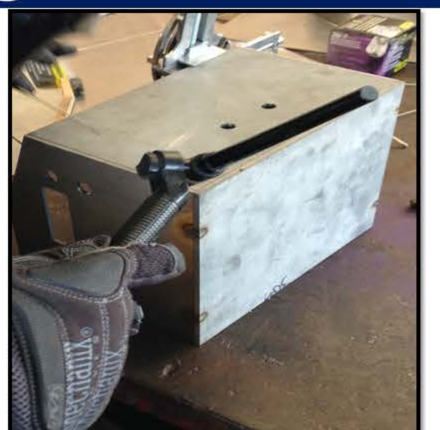
Frame TIG welded using 308L filler material
