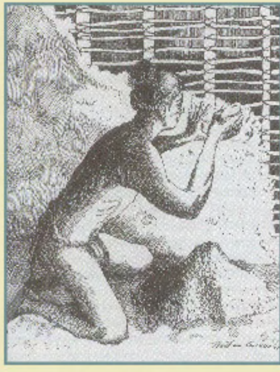
Applying daub (clay with Spanish moss) to wattle to create a wall.
